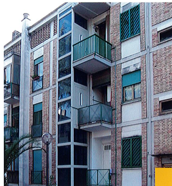
Outdoor installation in a condominium (Italy), structure with glass mirror cladding.
