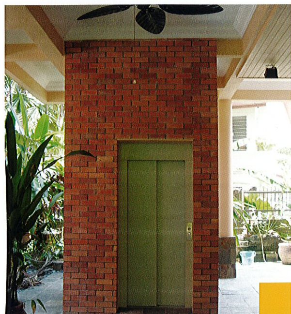
Installation in a private house (Malaysia), finishing in colored stainless steel, automatic 2 panels telescopic doors.
