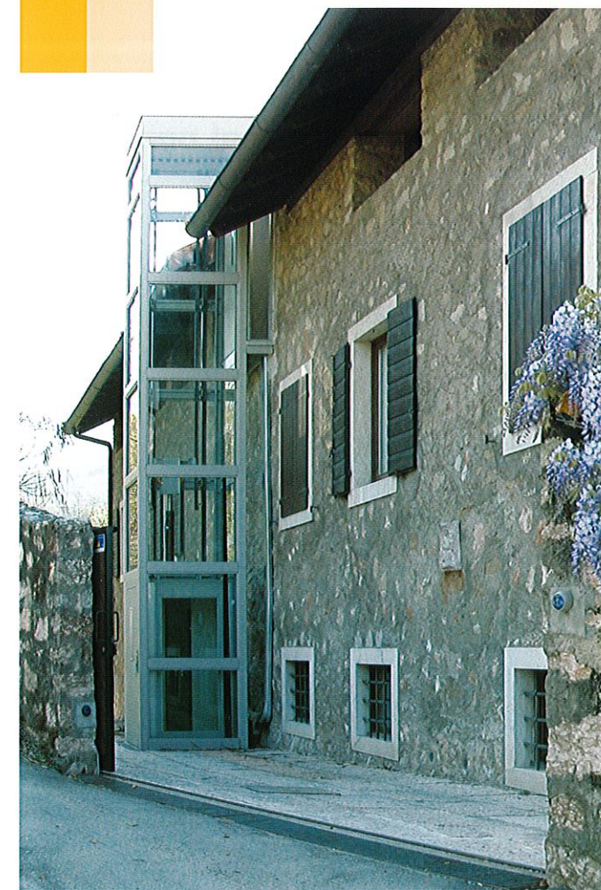
External installation in a private house (Italy), structure supported frame in stainless steel with glass cladding.
