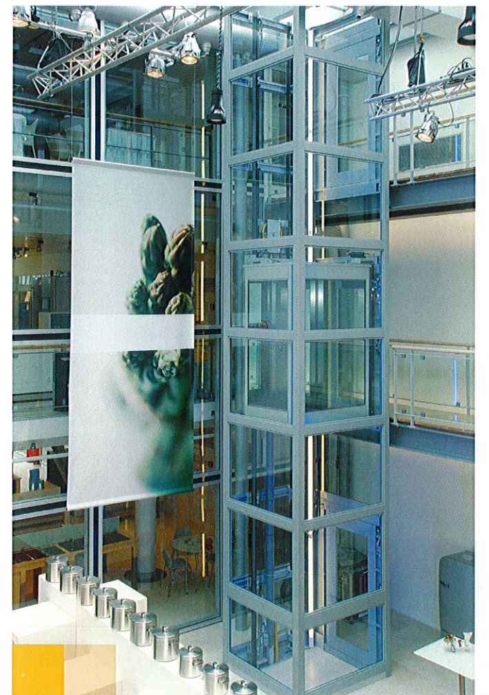
Indoor installation in a company (France), with structure supported frame in stainless steel and glass cladding.
