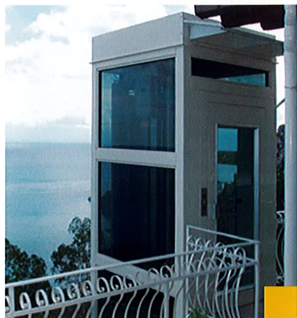
Installation in a private house near the sea (Italy), structure supported frame in white steel sheet and glass cladding.
