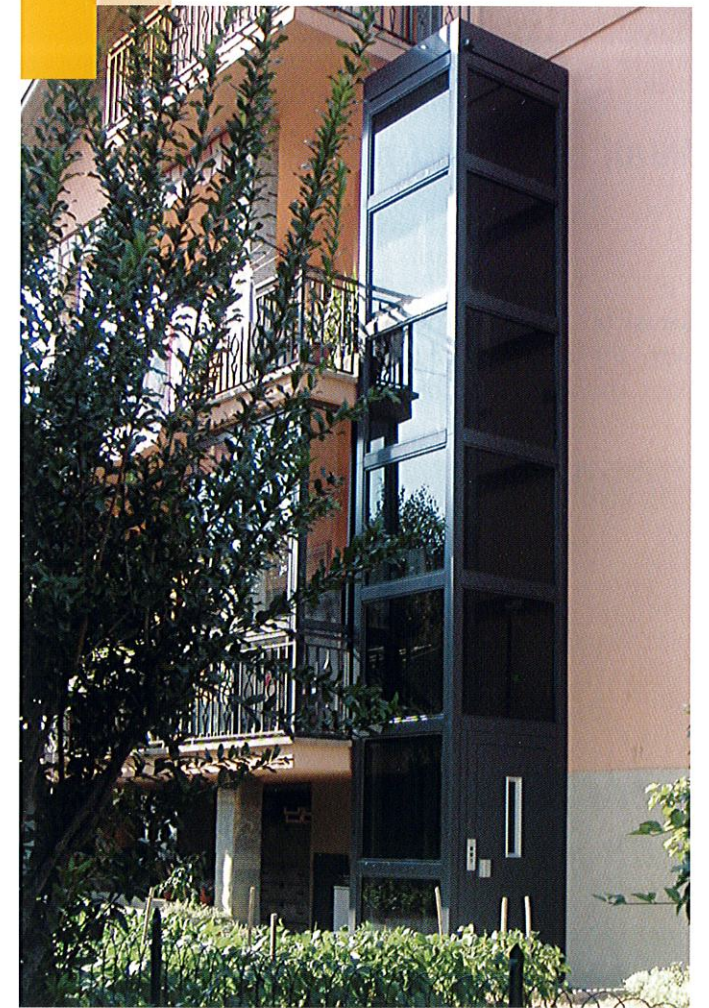
External installation in a condominium (Italy), finished in painted sheet steel and structure cladding in smoked glass.
