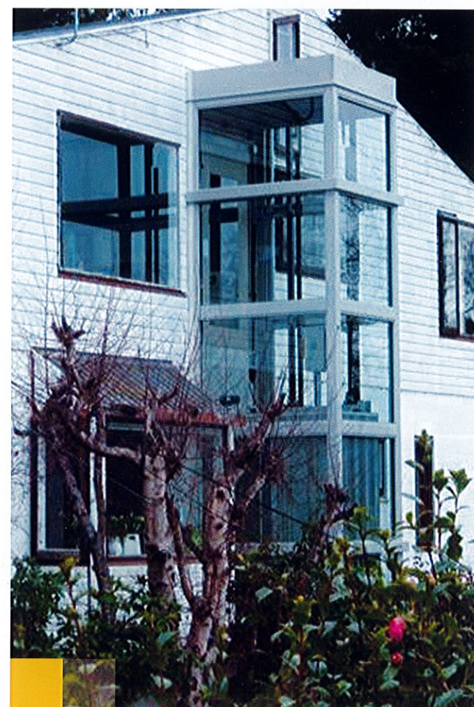
Outdoor installation in a private house (New Zealand), structure supported frame in stainless steel and glass cladding. Level is the ideal solution to move people easily, even for short distances.
