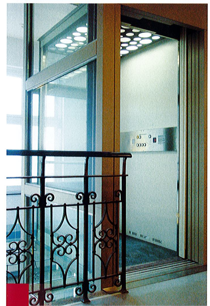
Installation in a public building (Italy), stainless steel structure with glass cladding, car with panoramic wall, 2 panels automatic telescopic door, car walls finishes in white skinplate.
