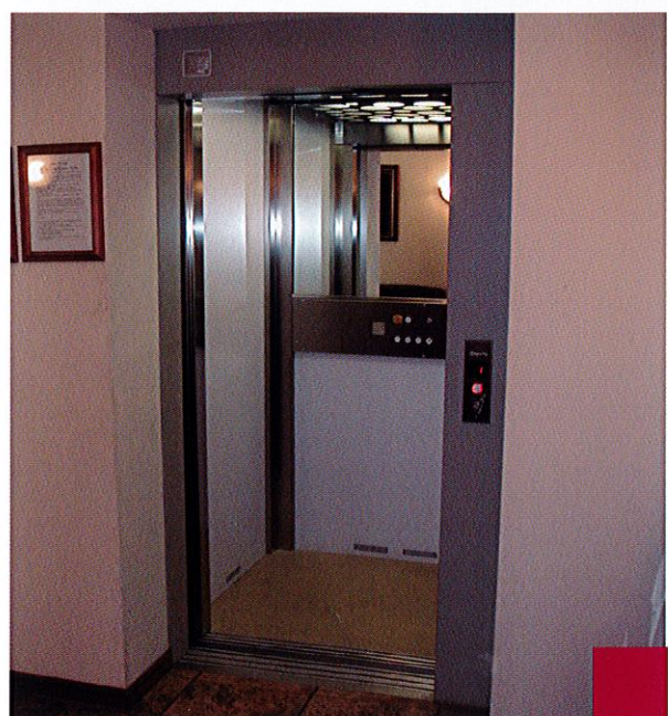
Installation in a hotel (Russia), car with skin plate panels, push buttons and car profiles in stainless steel, half wall mirror.
