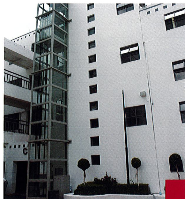
Outdoor installation in a condominium (Mexico), structure cladding in glass. Thanks to the structure supported frame, the lift can be installed also without a dedicated shaft.
