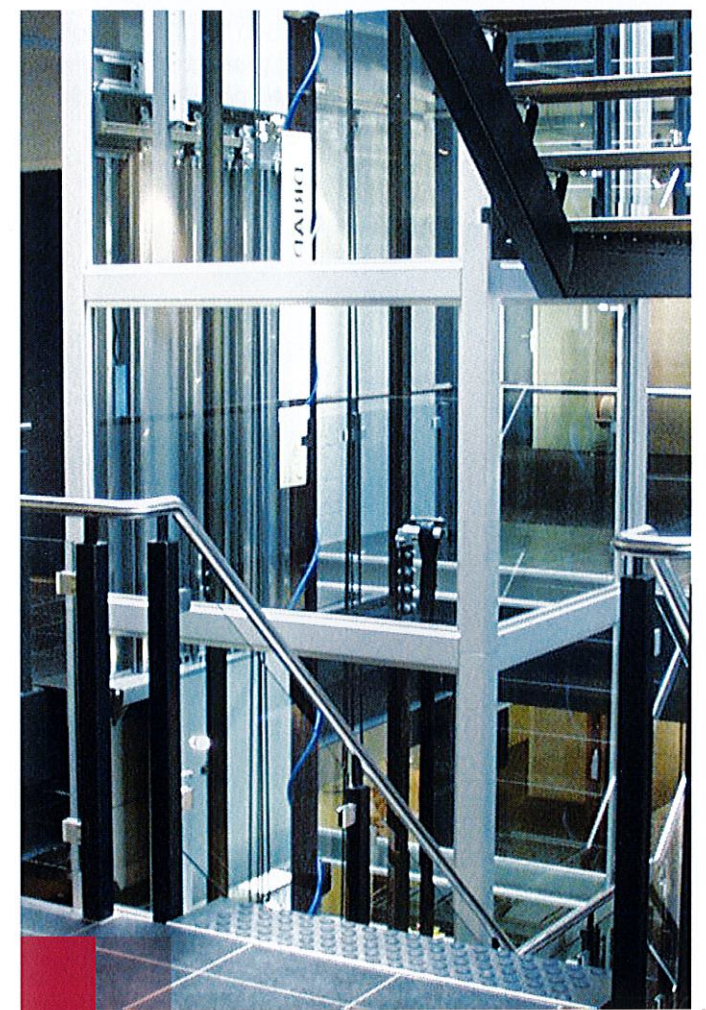
Installation with structure supported frame in a company (The Netherlands), finishes in skin plate and glass cladding.
